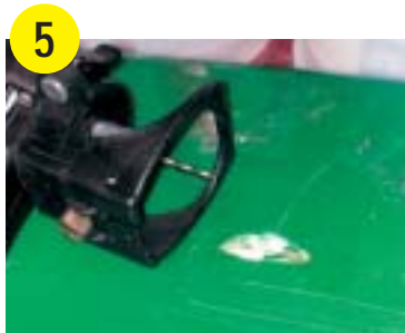
5 A rotozip or dremel can be used to remove the damaged fiberglass.
