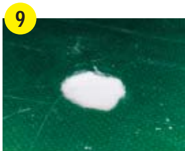
9 Pour the "resin foam" into the hole just to the bottom of the fiberglass skin. Resin will gel in about 10-15 minutes.
