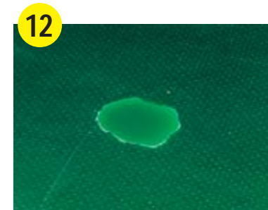
12 Buff out the area with 3M fiberglass restorer or any rubbing compound and repair is complete. Color match here is off, but the repair is undetectable to the touch.
