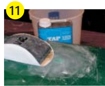
11 Once cured, sand smooth with successive or its of sandpaper.
